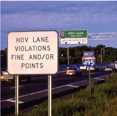
Future I-495 Express Lane, Virginia
